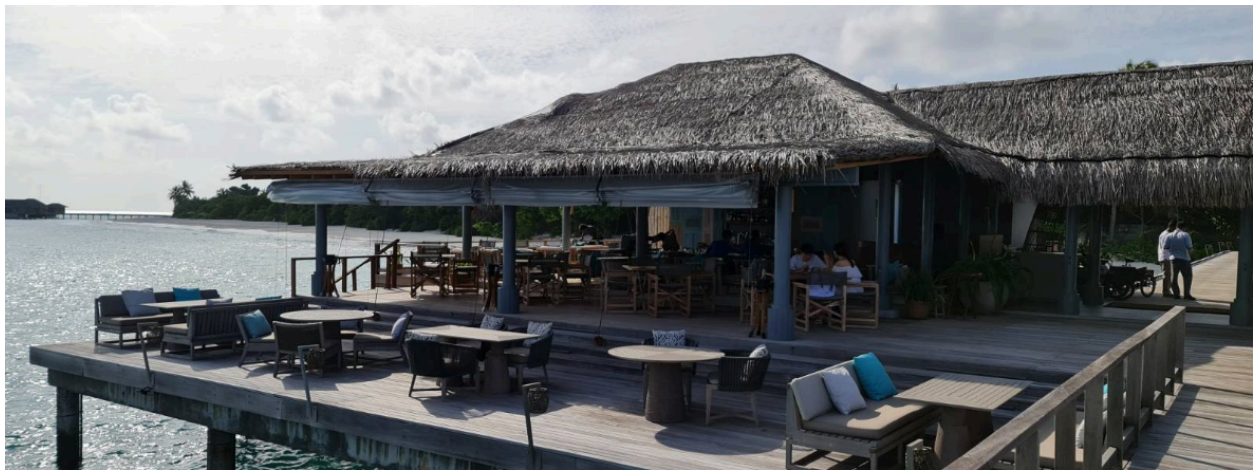
Structural capacity assessment of piles at overwater Lagoon Bar at Vakkaru Maldives Resort (2022)
