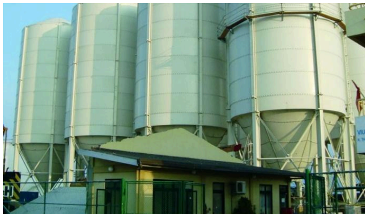
Concrete foundation for Cement Silo for Villa shipping and Trade Pvt Ltd.
