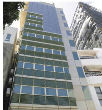
Existing structural conditions assessment of ADK Tower monitoring during Holiday Inn Hotel Construction
