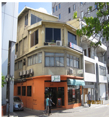
Existing Structural Conditions Assessment of H. Karankaa Villa, Male
