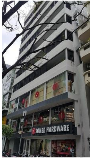
10-Storey development at H. Emboogasdhosuge (Completed)
