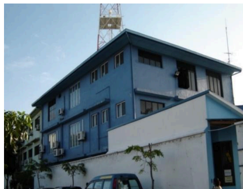
Existing Structural Conditions Assesment of TVM building, Male
