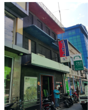
Existing Structural Conditions Assessment of Olympia Building, Male
