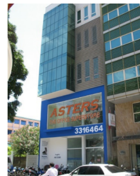
Existing Structural Conditions assessment of Aster Building, and Monitoring during Holiday Inn Hotel Construction
