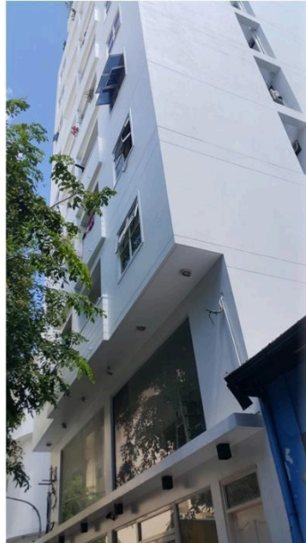
G. Quest, residential commercial building
