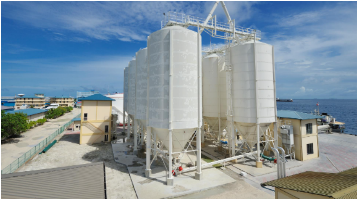
Structural design of foundation for cement silos (at Thilafushi reclaimed area) for Villa shipping and Trade, Maldives
