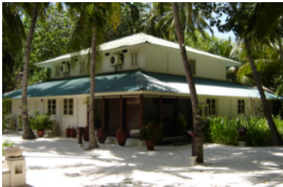
Existing Conditions assessment of Administration & Finance building at Banyan Tree Resort.
