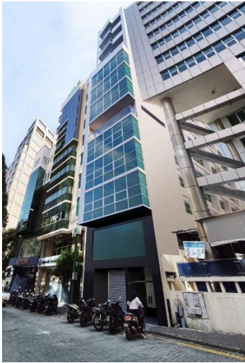
15-Storey development at H. Athireege (construction ongoing)
